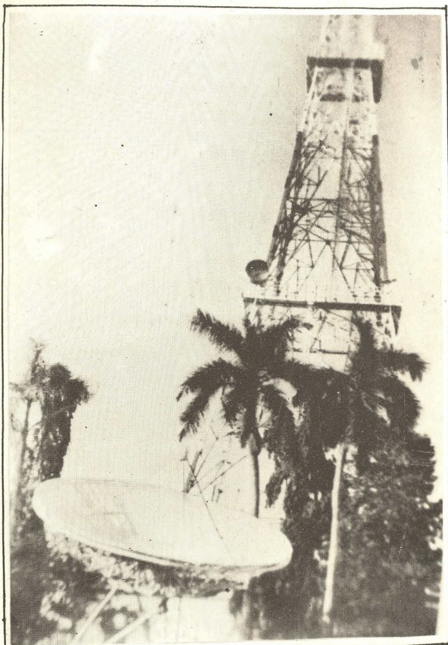
Antenna and the Transmission tower of Doordarshan Kendra, Cuttack
